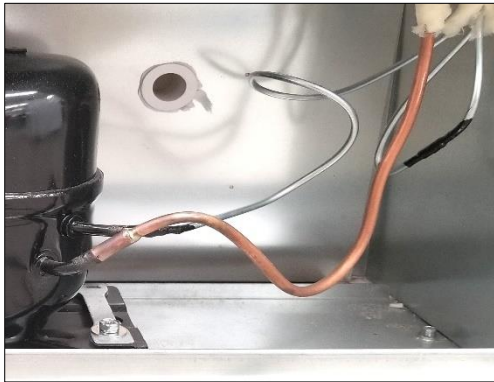
Figure 7. Access Port External View
